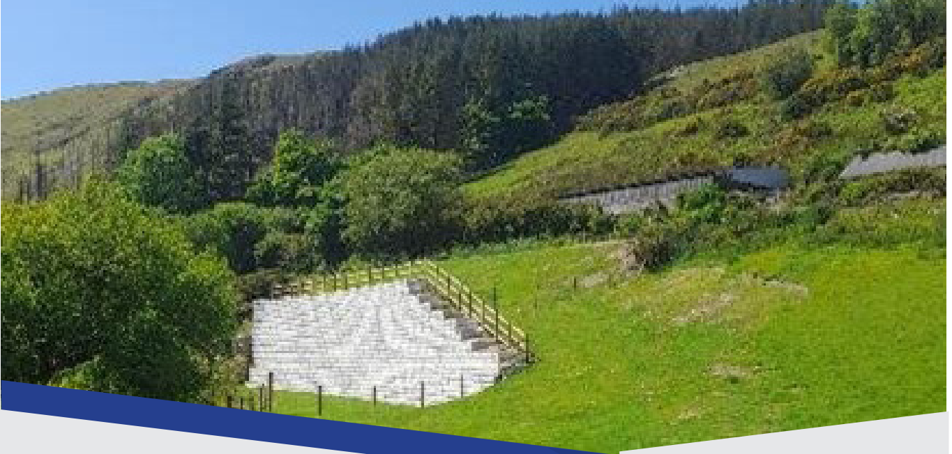
Retaining Wall at Gleann Gheis
