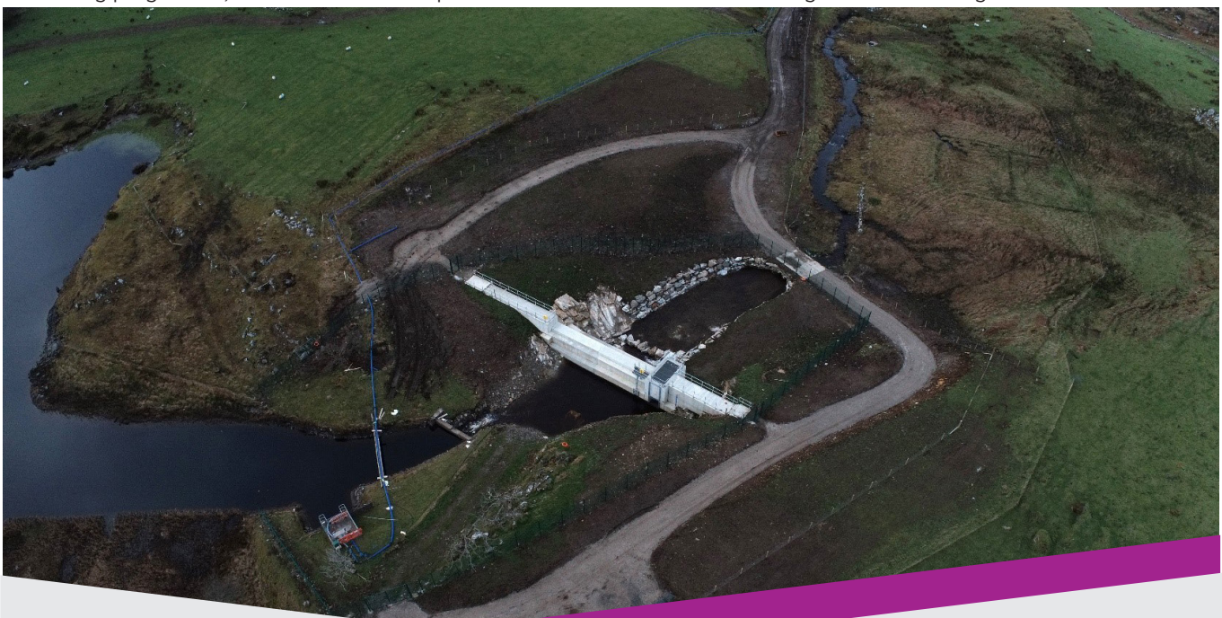
Aerial photograph of the dam at Lettermacaward WTP
