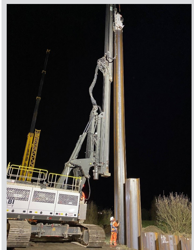
Piledriving works on the N56 Letterkenny Four Lane
