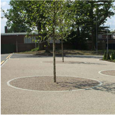
Figure 27- Resin bound gravel is a flexible, permeable material, making it well suited for infill of tree pits.
