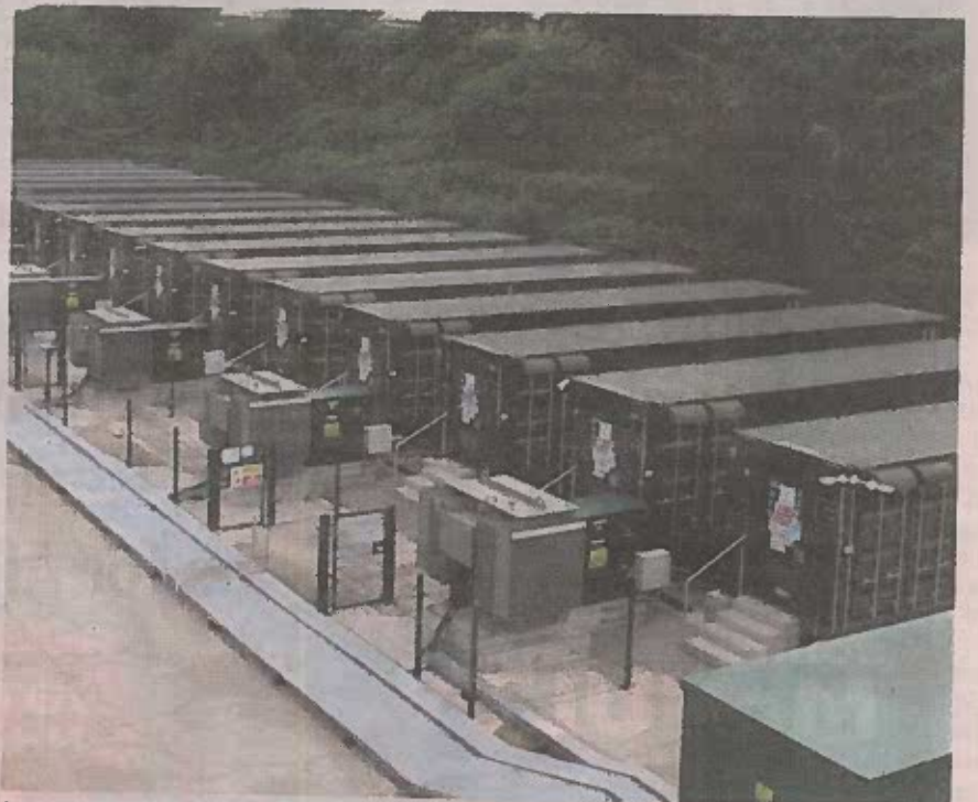
An example of 16 skids while 48 were planned for the Ballyshannon development
