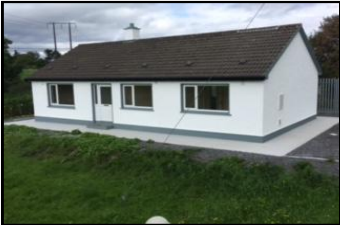
Dwelling refurbishment in Ballyshannon
