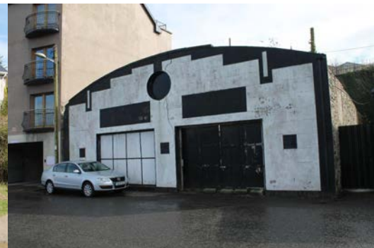
Garage, Shore Road
