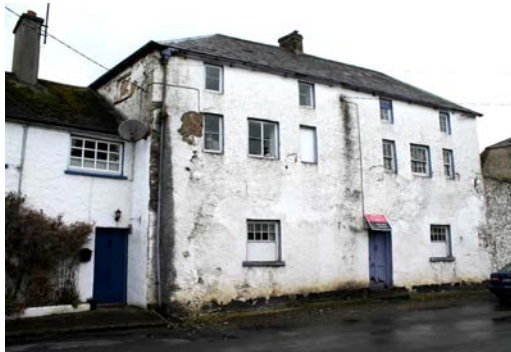
former Guild Hall, Castle Street – NIAH 40800416
