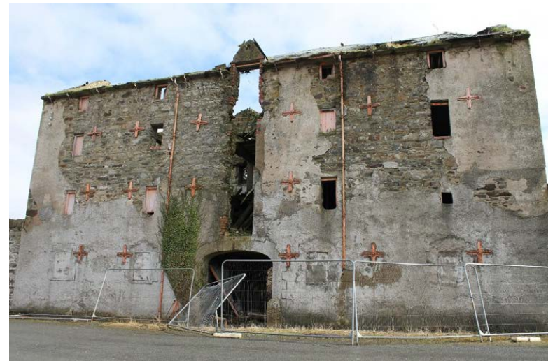
Warehouse, The Quay - NIAH
