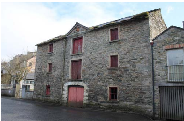
Warehouse, Shore Road –RPS & NIAH 40800412
