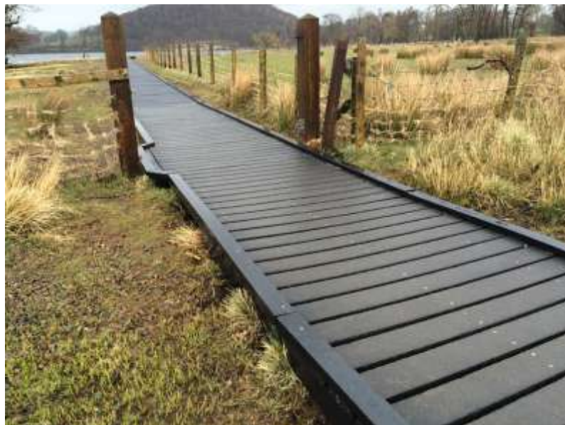
Example of Recycled Plastic Boardwalk
