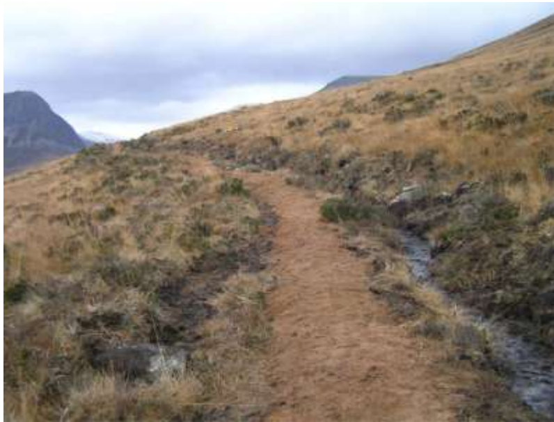
Example of raised aggregate path in upland blanket bog in Scotland
