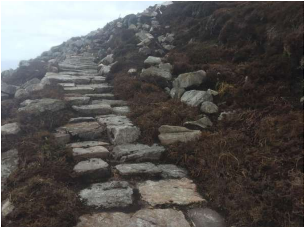
Weathered quartzite stone pitching on Sliabh Liag, Co Donegal. The path looks natural and 'old,' and very much in keeping with the surroundings
