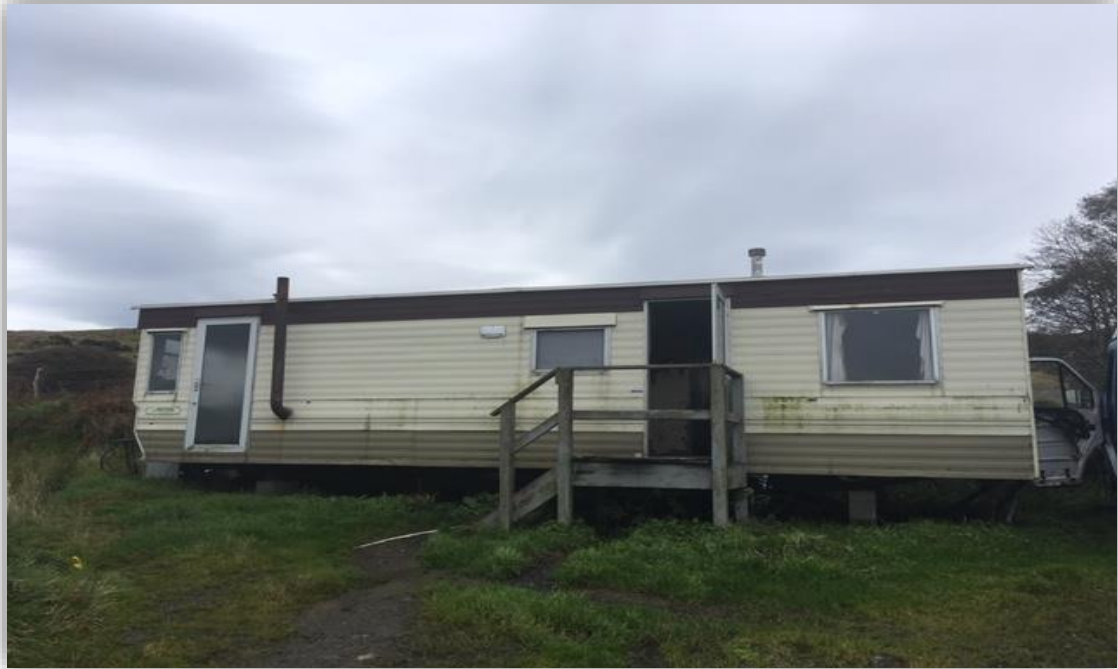
Cashel Ardara Single Unit accommodation replacement - Before
