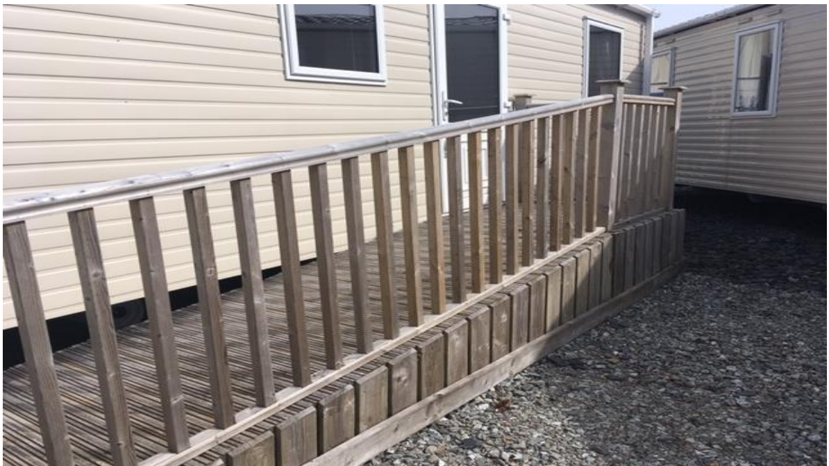
Miscellaneous Project Example 2 – Ramp to mobile home
