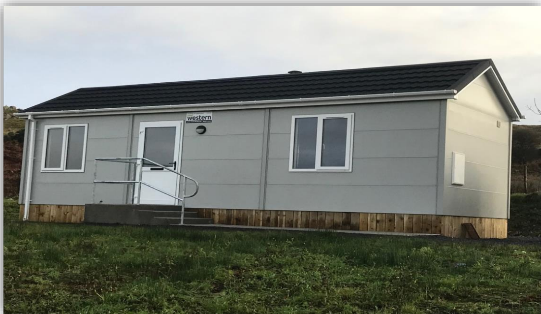
Cashel Ardara Single Unit accommodation replacement – After
