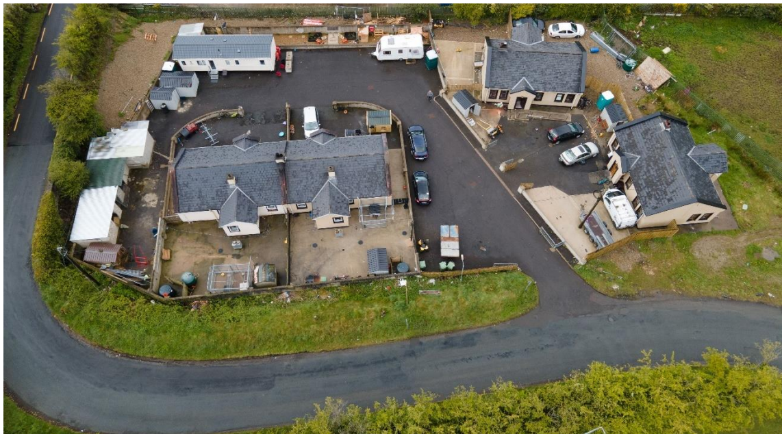
Cullion Road Group Housing scheme, Letterkenny
