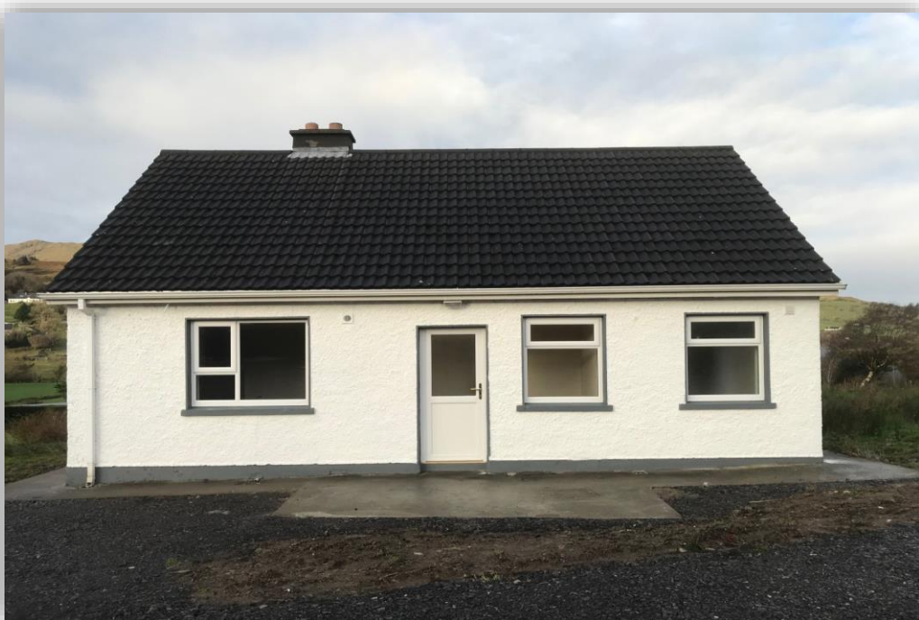
Cashel Ardara Dwelling Refurbishment - After
