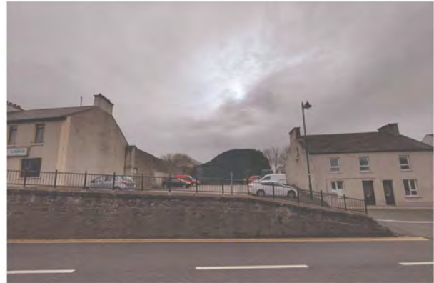
Existing Cope Yard, Creelough © Arup
