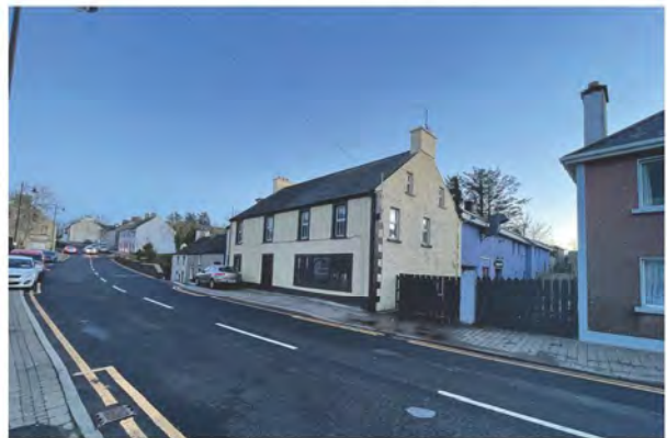
Derelict building along Main Street, Creeslough © Arup
