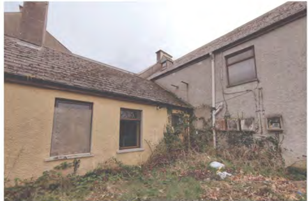
Derelict building and court along Main Street, Creeslough © Arup
