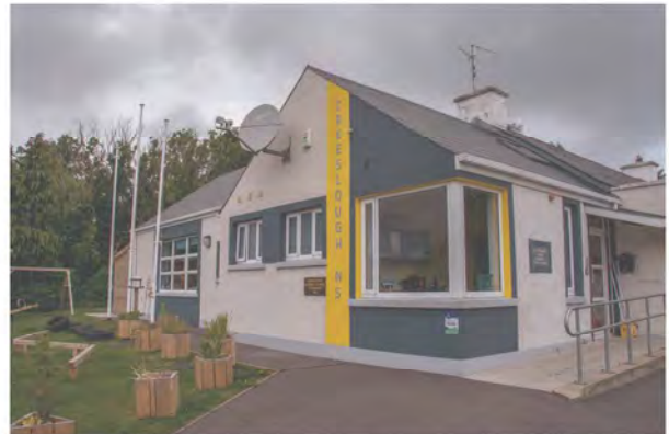
Creeslough National School © Arup
