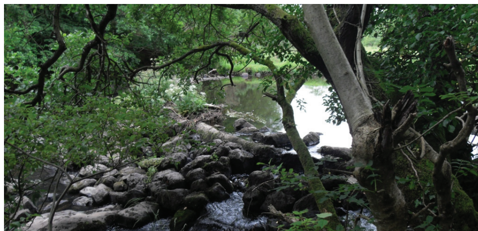
Weir on the Ballinderry River
